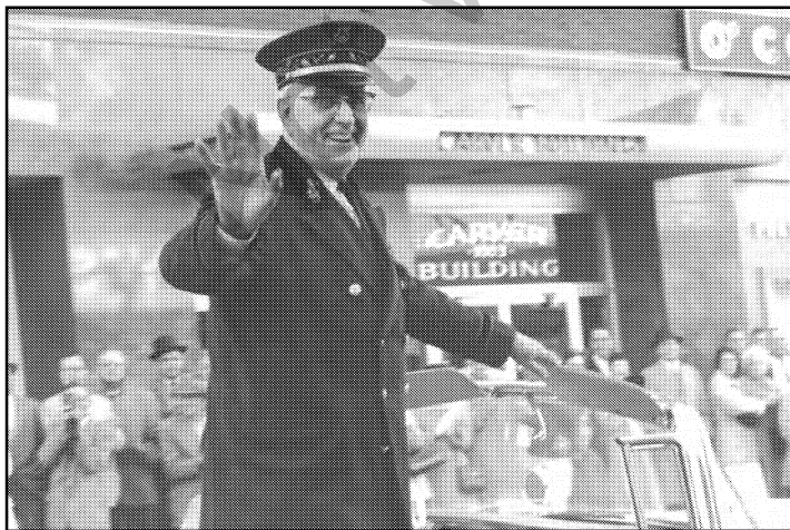
A famous photograph of Karl L. King, riding in a convertible down Central Avenue in Fort Dodge, Iowa, around 1960. The Carver Building in the background still stands, although the overhang with the building's name is now gone. On the opposite side of this building was the K. L. King Music House, at 1012 Central Avenue.
